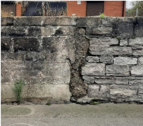
**Fig. 4.2.27** - Modern section rebuilt with concrete blocks
