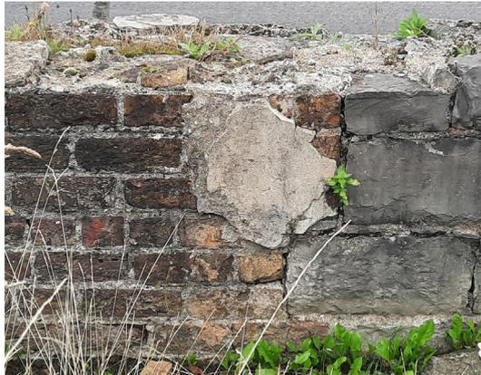
**Fig. 4.2.28** - Typical wall top treatment to low section of wall
