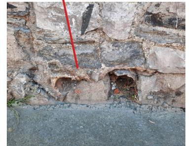
**Fig. 4.2.24** - Clay pipe outlets
