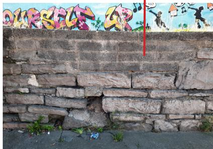
**Fig. 4.2.22** - Concrete blocks replacement at upper section. Pointing washed out at lower section and loss of a few facing stones
