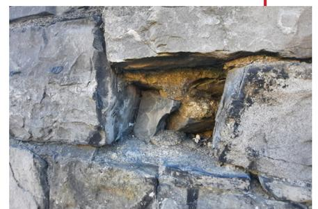
Fig. 4.2.25 - Loss of facing stone
