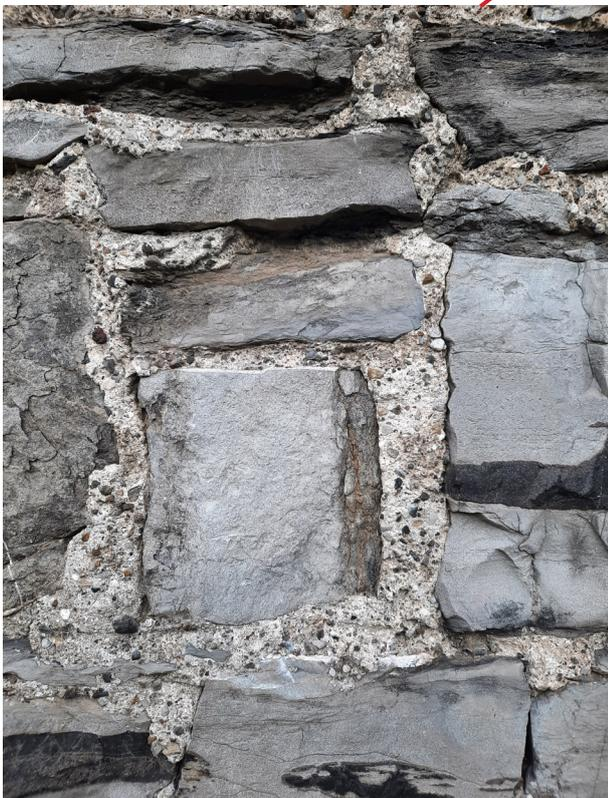
**Fig. 4.2.15** - Typical lime mortar found along lower section of wall
