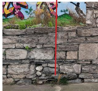
**Fig. 4.2.23** - Loose masonry at lower section
